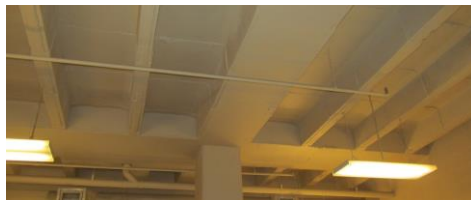
Figure 2 - Pan and Joist Floor Construction
