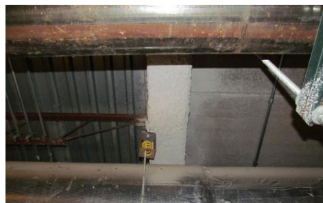
Figure 6 – Penthouse roof interface between metal deck and concrete plank
