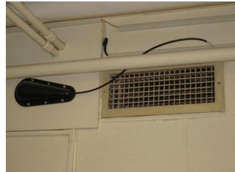
Photo 10: Internal Distribution Antenna
