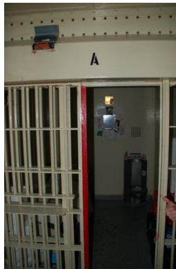
Photo 2: Cell front sliding device
