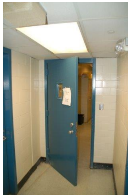
Photo 6: Door at smoke barrier
