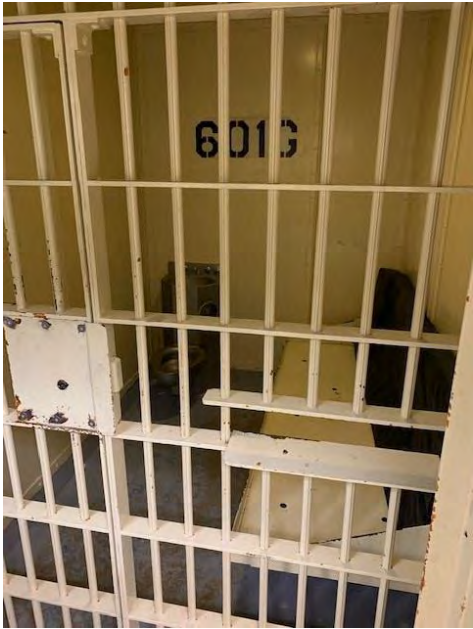
Existing CCB Cell Blocks
