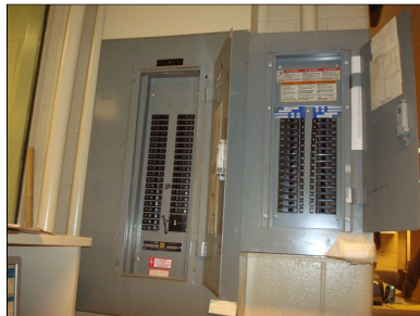
Panels 7/X and 7/XE (Seventh Floor West) Installed in 2001.
