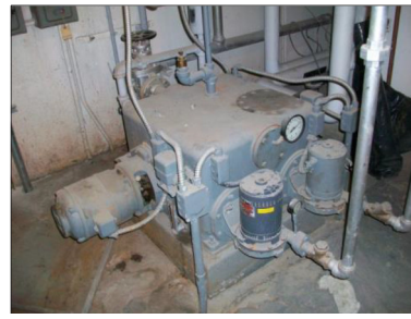
Steam Condensate Receiver and Pump
