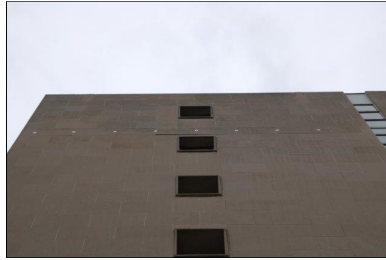
South Elevation Showing Repair
