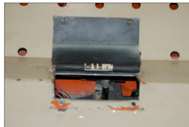
Sliding device manual release
