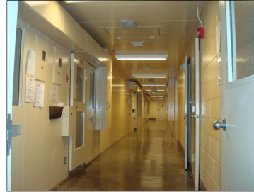
West wing metal panel cellblock fronts
